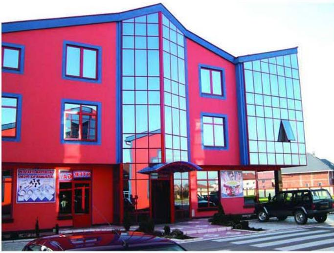
Modern curtain wall system with cell structure and 16mm clearance between its element. The system has the following special features:
