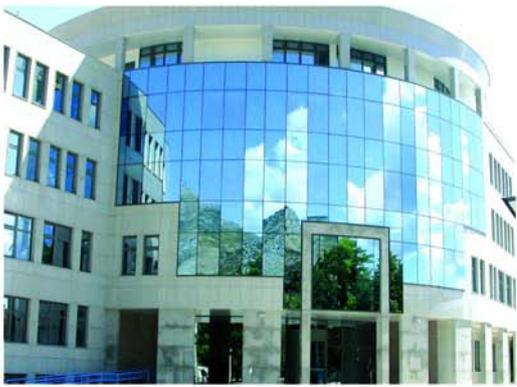
The system uses the same profiles and components as the M3. The main difference is that the aluminium is not visible from the outside thus the glazing surface seems uniform.
